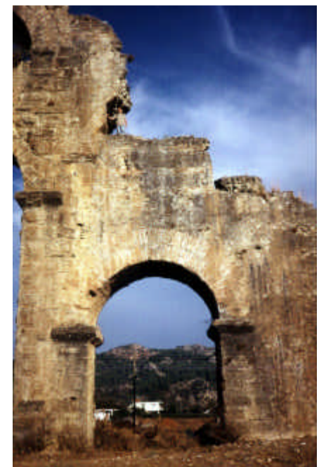
Detail of north tower Detail des Nordturmes
